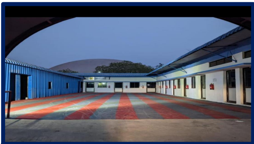
Building Renovation @ DVM Kadapa
