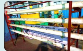
Hydroponics System Under Construction @ DVM Rajgangpur
