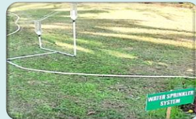
Water Sprinkler System @ DVM Chirawa
