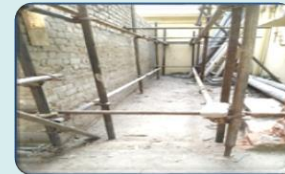
Bamboo Skill Center and Combo Bio Toilet under Construction @ DVM Rajgangpur
